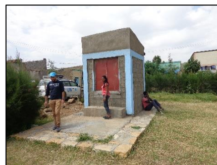
Picture 1: Water kiosk, Wukro
